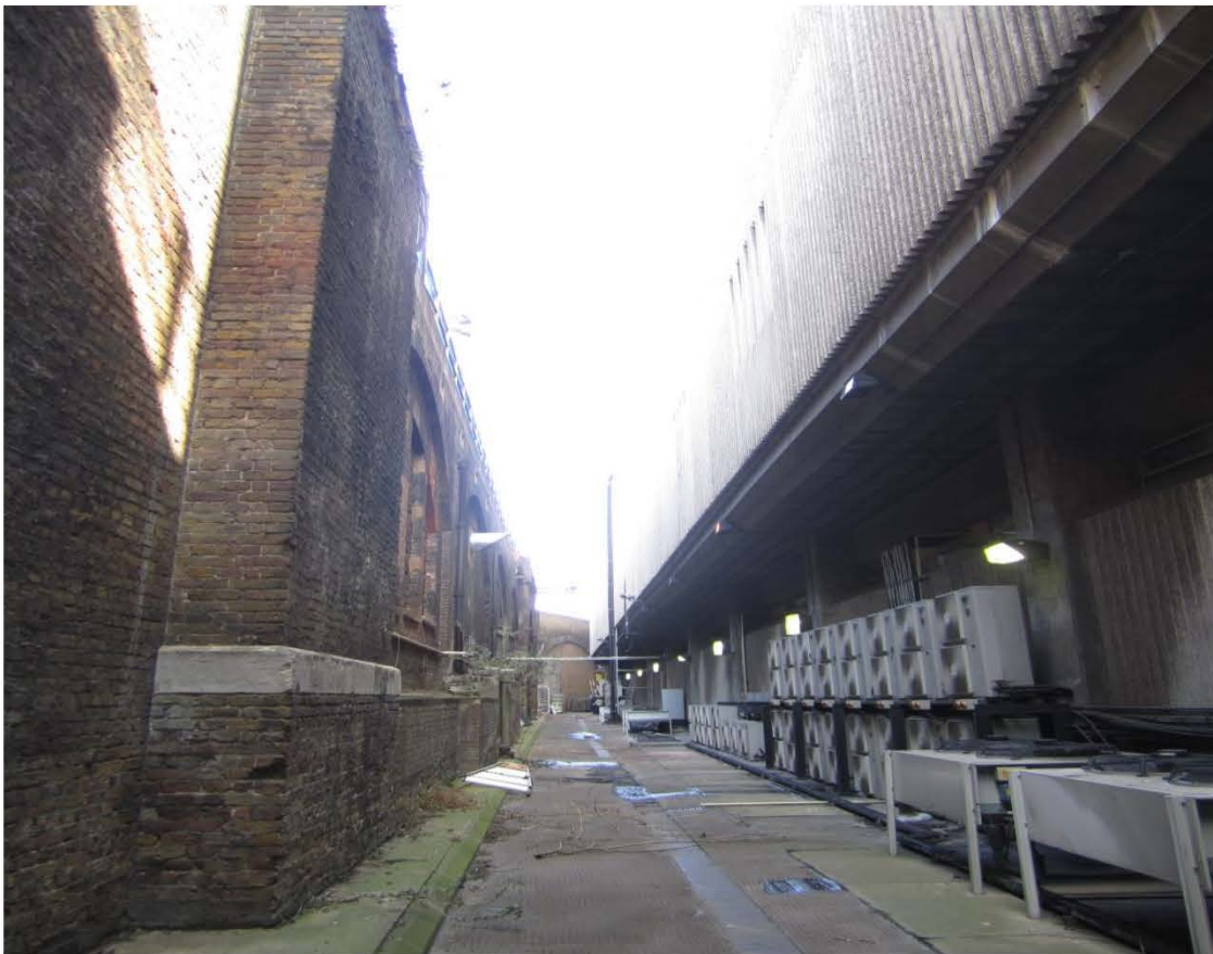
Photo 2 – Passage between Viaduct and Sampson House
