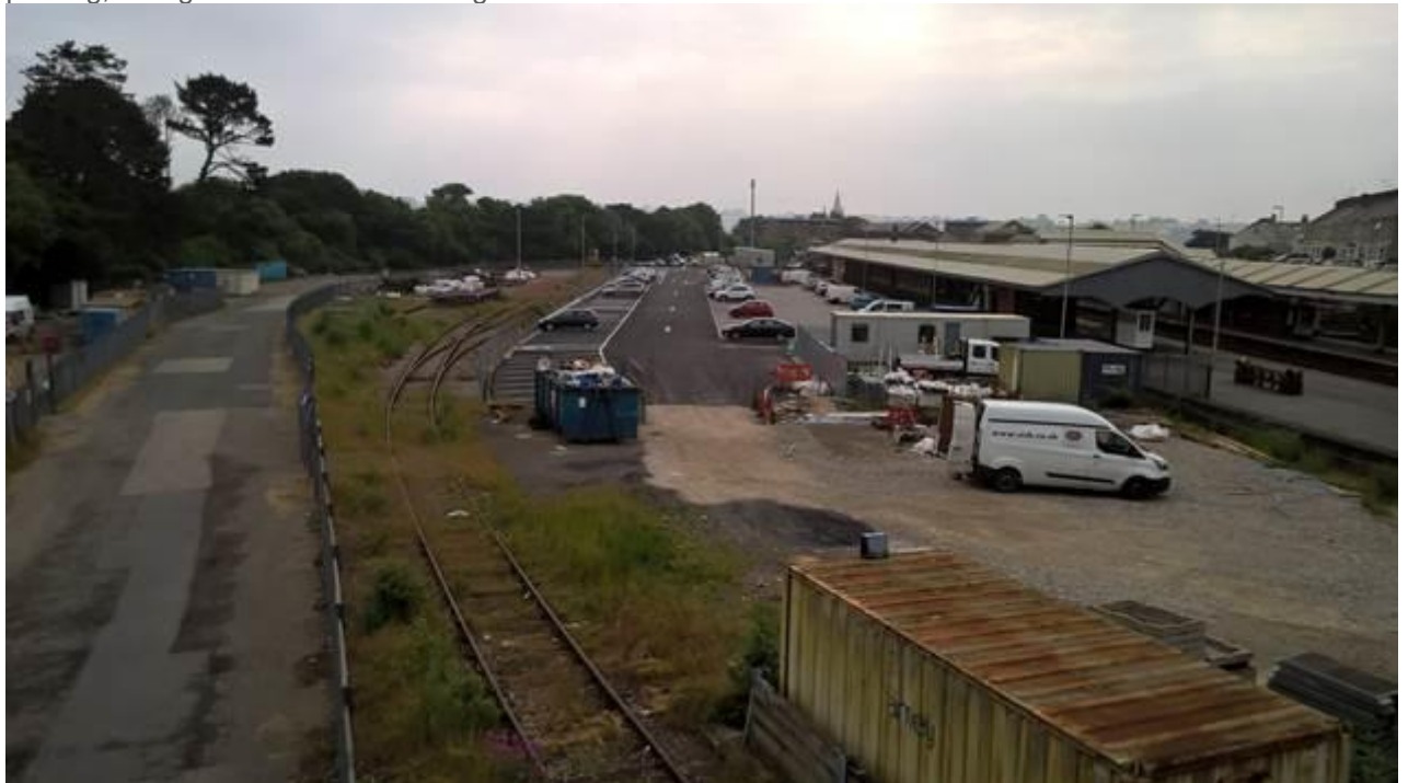
View from the footbridge looking East towards the station showing the newly improved passenger parking, sidings & NR informal storage.
