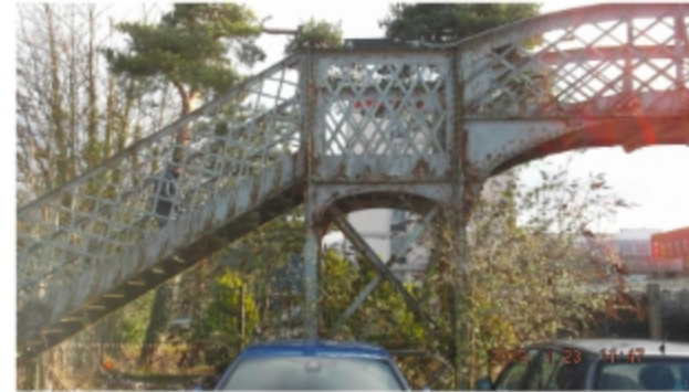
Detail of pedestrian bridge and intermediate landing
