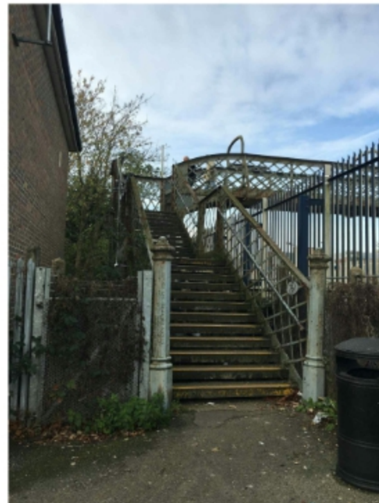
Pedestrian bridge as it lands on East Park
