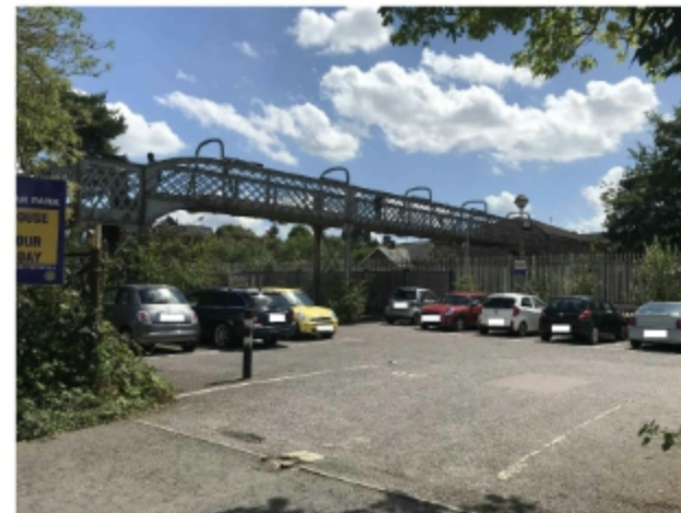
Pedestrian bridge from Star Park Car Park
