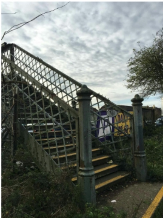
Pedestrian bridge as it lands on Station Way
