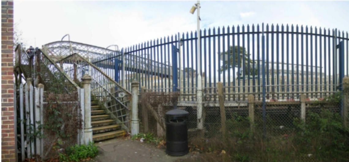
Pedestrian bridge from East Park
