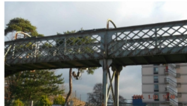
Detail of pedestrian bridge and intermediate support
