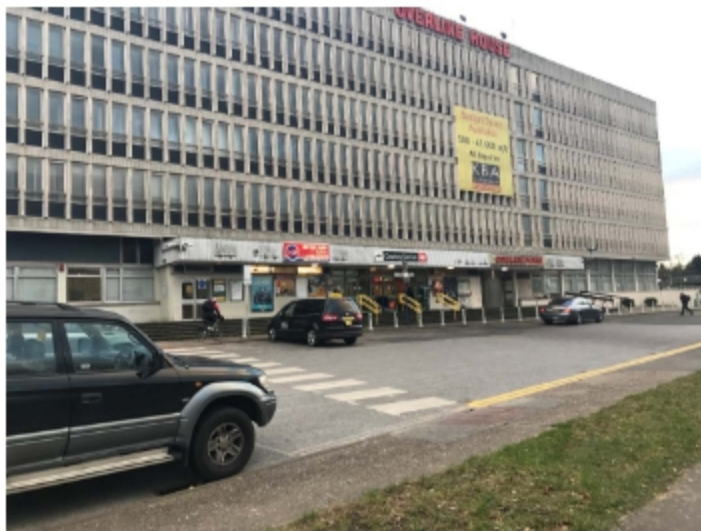
Photograph 2 - Overline House showing location of Station at ground floor with existing office entrance to right, station forecourt and current drop off and taxi rank.
