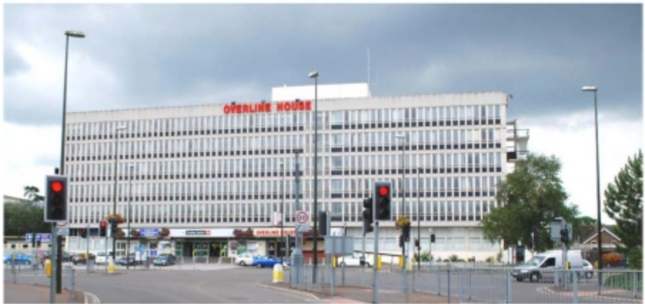
Photograph 1 - Overline House with station on ground floor viewed from Friary Way
