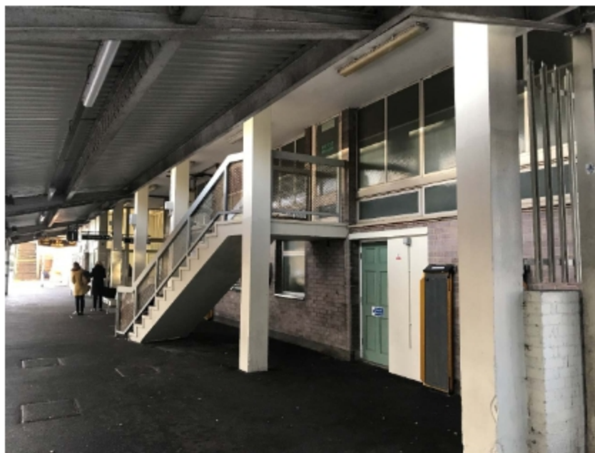
Photograph 4 – Existing fire escape from Overline House onto station platform
