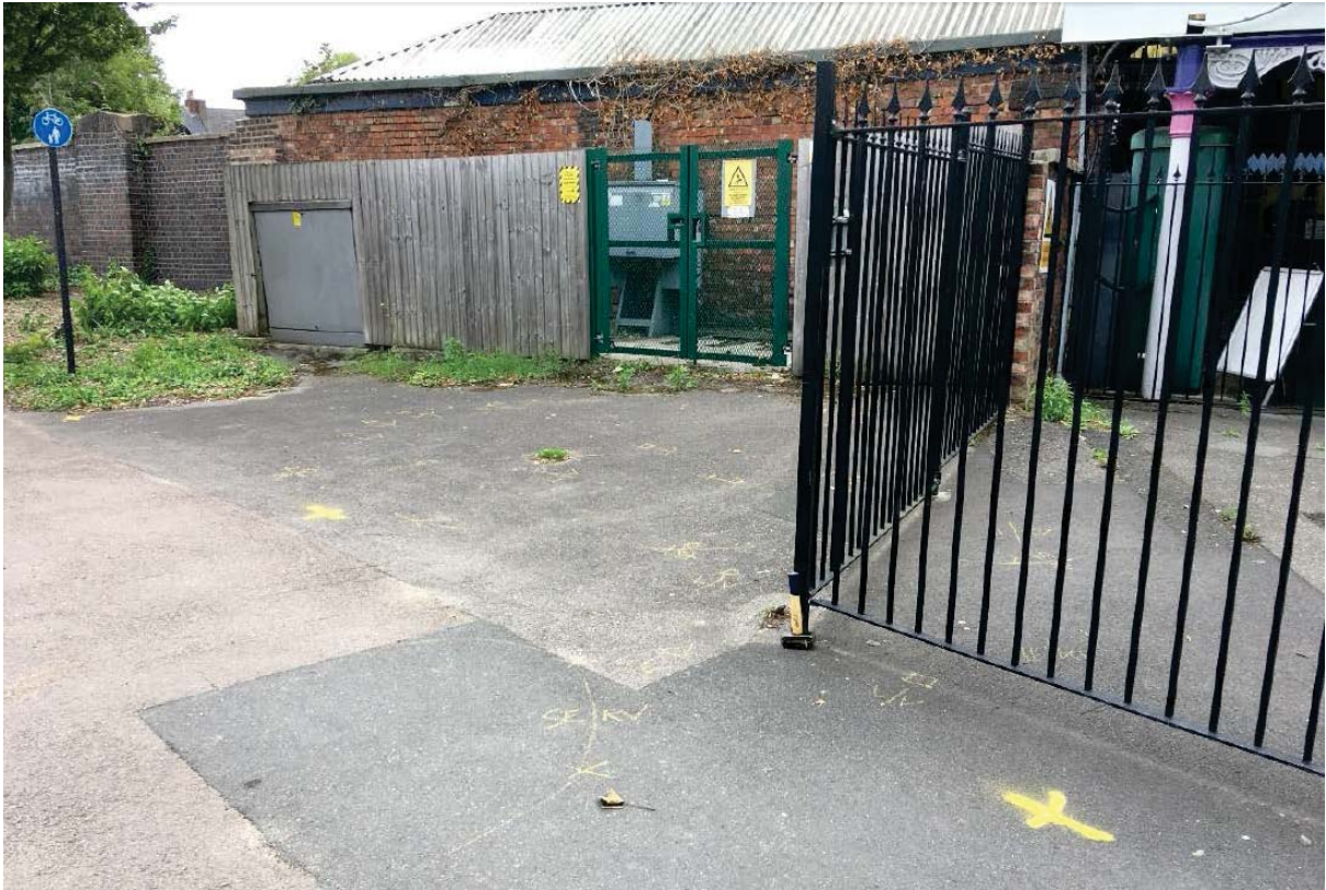
Above: Looking north-east (existing sub-station on right of photograph). Taken: August 2019
